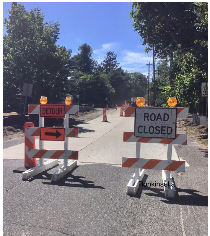
Beaver Dam Road Construction Sign By Ron Kinsella
