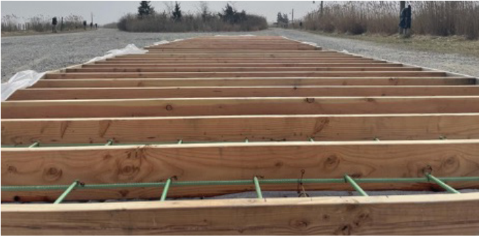
Ramp shell waiting for concrete.
