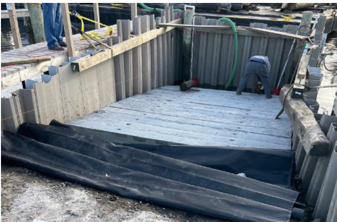
Ramp Install, Spring '22
