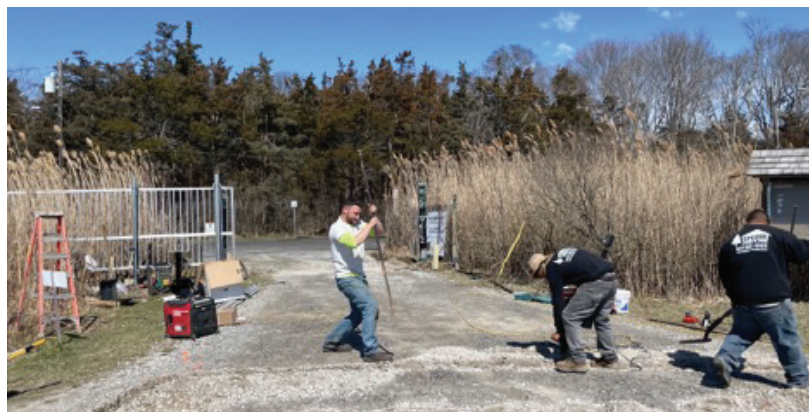
Fence installers preparing the ground sensor for the new automatic gate.
